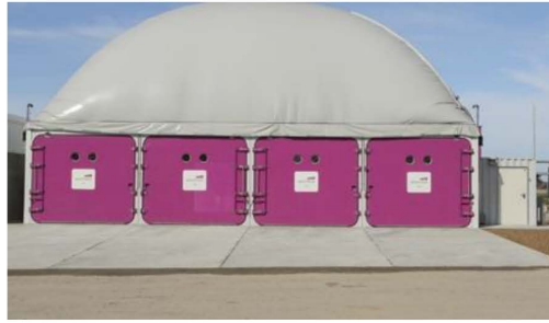
Major step towards waste decentralization: Small-scale dry-waste ADs like these are expected to become widespread in the US over the next decade.
